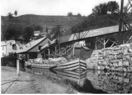
FIG. 11—Loading dock of the Consolidated Rosendale Cement Company along the Delaware and Hudson Canal at Binnewater Road in Rosendale. Notice the tramway directly above the canal barges. The cars on this tramway are loaded with barrels of natural cement produced from the Beech Mine along Binnewater Road. The structure built from dark iron girders at upper right is a footing for the Wallkill Valley Railroad Trestle over the Rondout Creek. This photograph was originally published by the Consolidated Rosendale Cement Company in a 57-page advertisement booklet in 1910 (collections of the Century House Historical Society).
