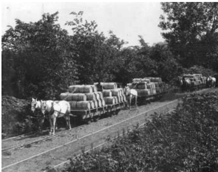
FIG. 12—Photograph of the horse-drawn railroad (ca. 1899?) that once transported natural cement manufactured at plants near Whiteport and Hickory Bush to docks at Eddyville along the Delaware and Hudson Canal (collections of the Century House Historical Society).
